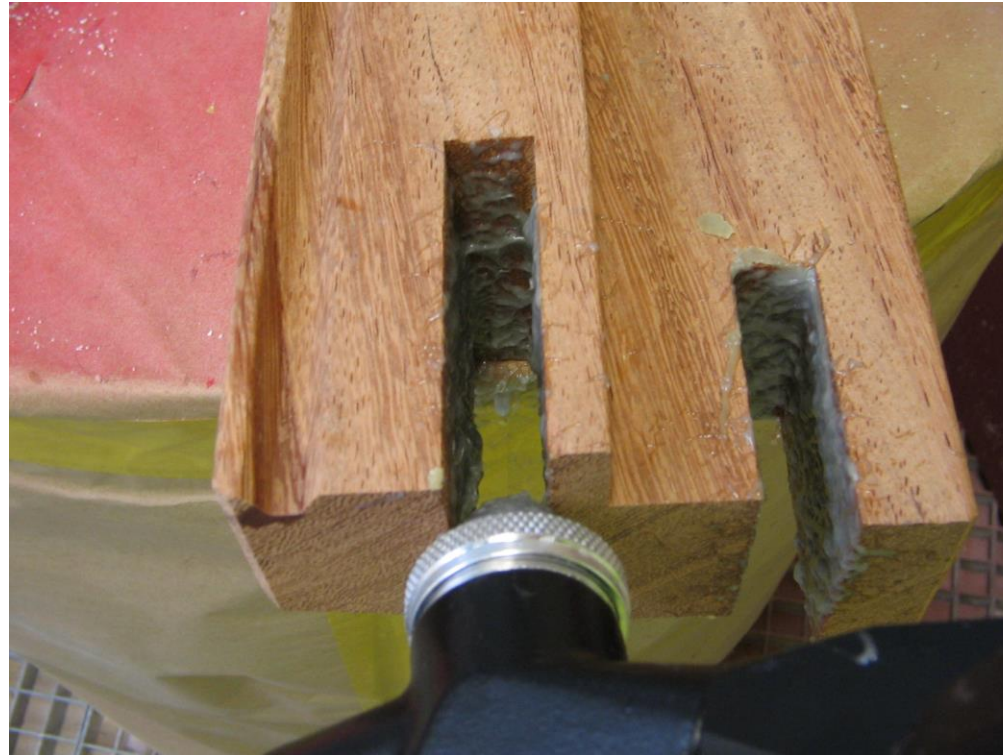
Application of Opti-Joint XP by spray-gun.
